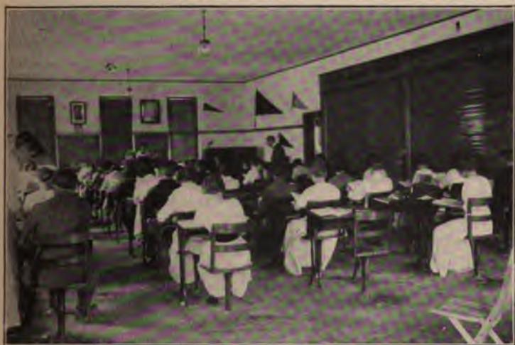
A movable partition for auditorium use, Cache La Poudre school
